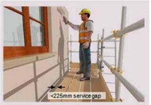
If the service gap is less than the width of a scaffold board, 225 mm, and there are no door or window openings through which an operative could fall, internal guard rails are not normally required.
