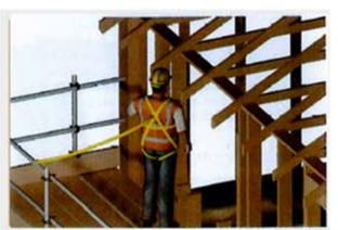
If an operative is required to work from an inner platform where the service gap exceeds 225 mm and presents the risk of injury, double guard rails should be provided at the inner platform edge connected with puncheors. Alternatively, a safe system of work must be employed that includes a full body hamess and restraint lanyard to prevent the operative falling from the inside open edge, unless another suitable means of protection is determined from the risk assessment.
