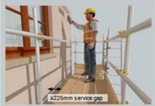
If the service gap exceeds 225 mm and presents a risk of injury, but not a risk of a person falling through the gap, a single guard rail may be required with a safe system of work that includes supervision, training and instruction
